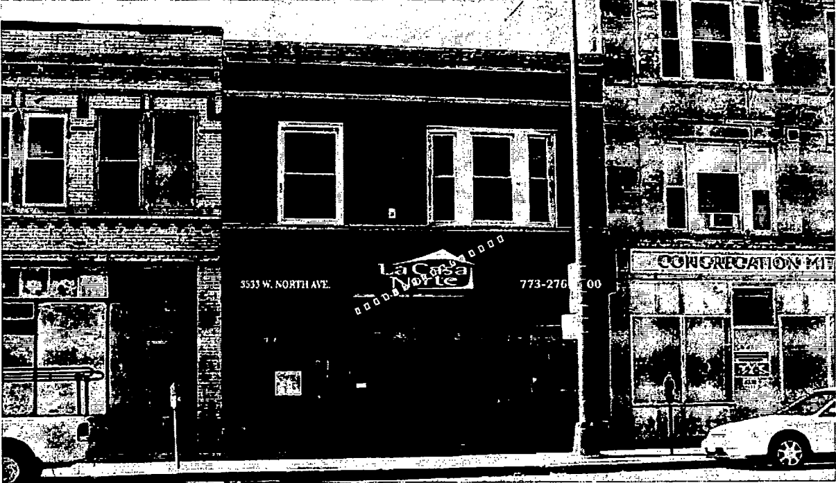
3533 West North Avenue
