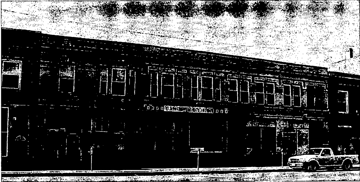
3527-3531 West North Avenue
