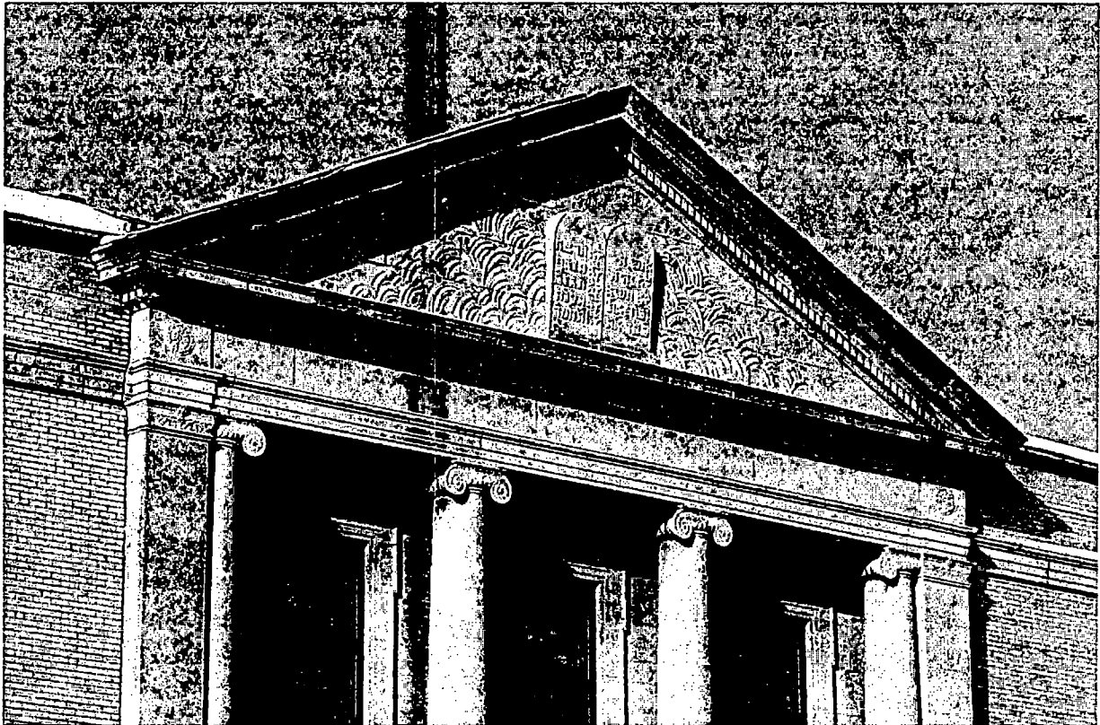
The (Former) Anshe Sholom Synagogue Building is built of yellow brick and gray limestone and designed in the Classical Revival architectural style. The main (Independence Blvd.) elevation has a large Classical-style "frontispiece" with gray limestone Ionic columns supporting a triangular pediment ornamented with tablets with Hebrew script.
